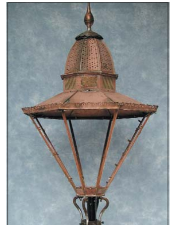
The finished refurbishment, reglazed and repainted, without the additional protection frame that was added later.
